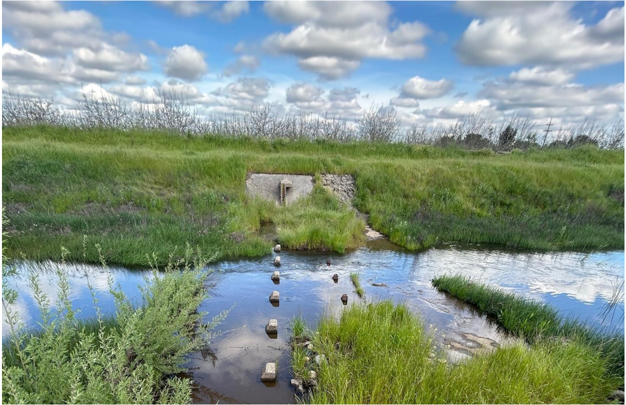
Bear Creek Dam near Harney Lane.
