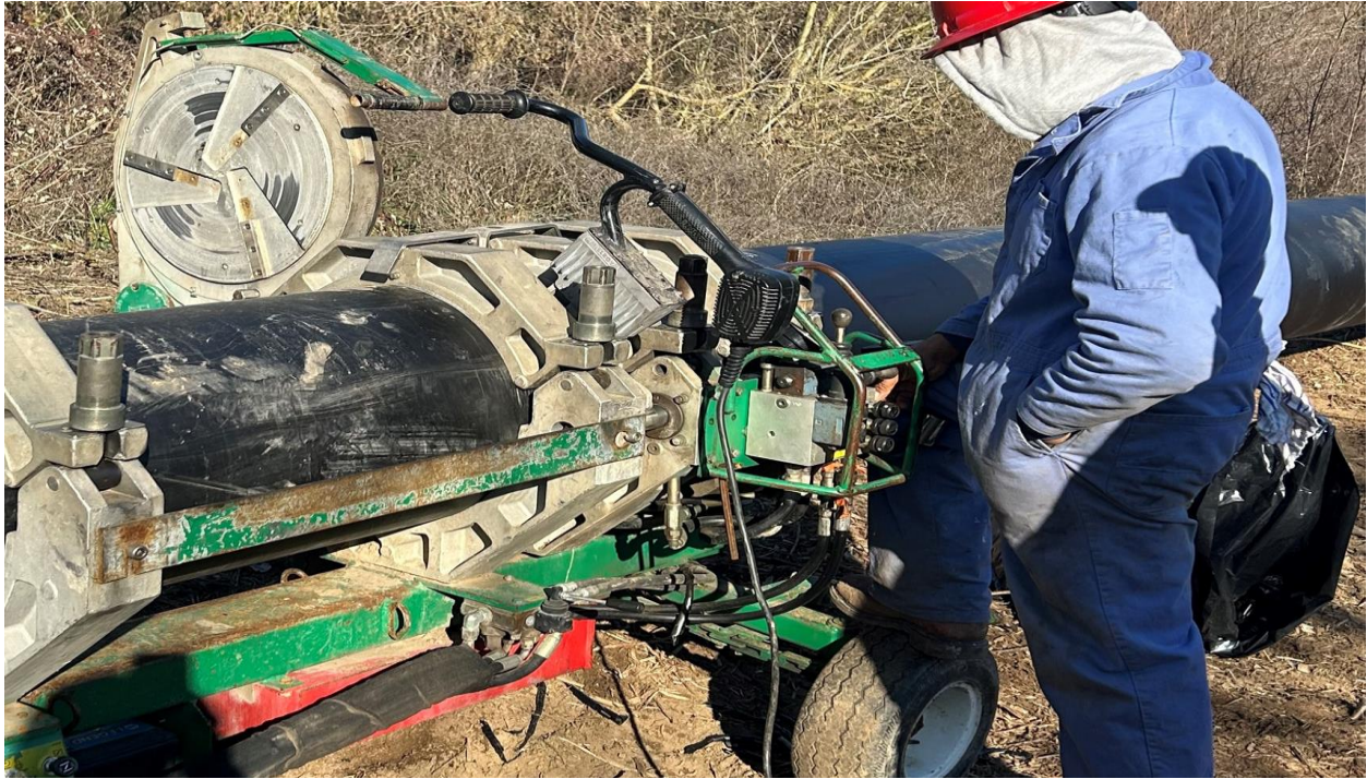
Pacific Southwest Irrigation Staff Fusing the HDPE
